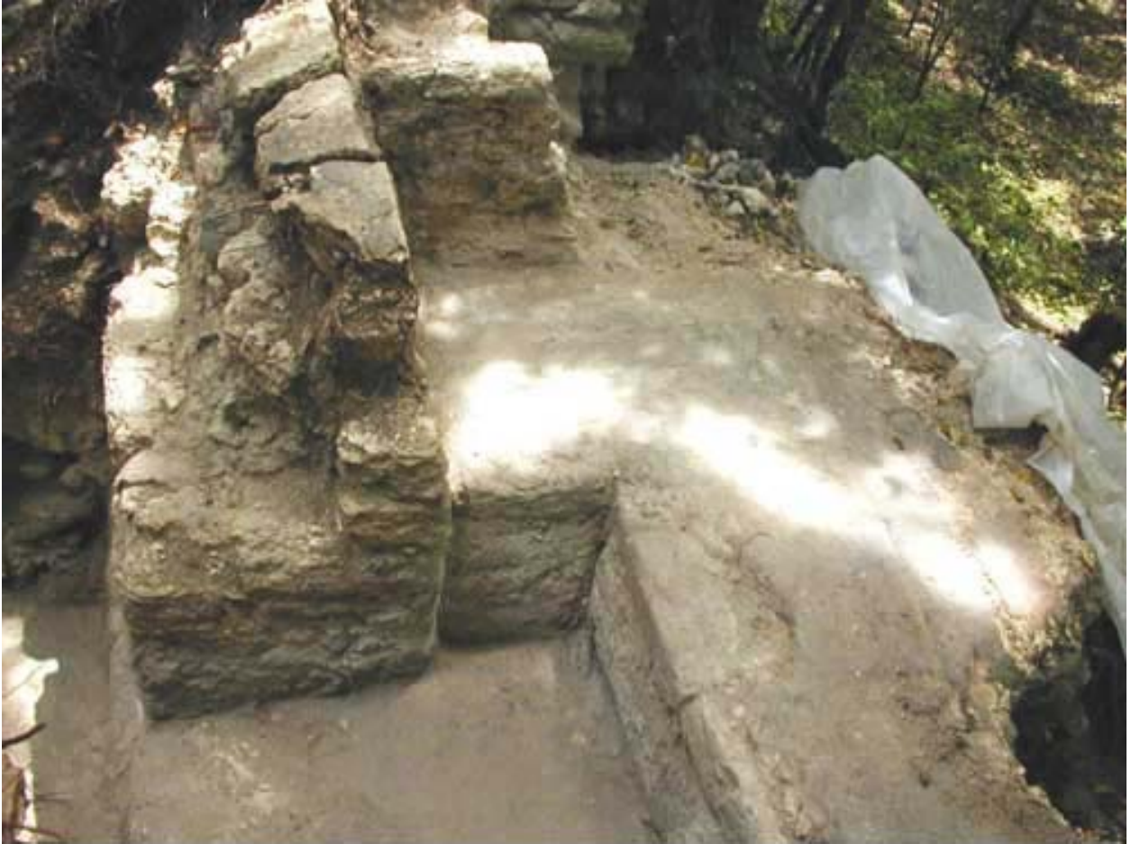
Figure 15. View of doorjamb, interior floor and bench of Str. 50. In the far right is a looters' cut.
