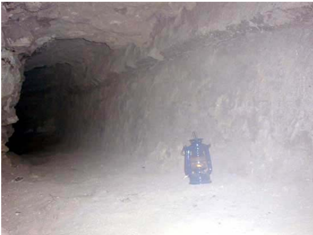
Figure 13. View of the tunnel in Str. 2, Group III A, exposing earlier stucco apron molding and bench façade.
