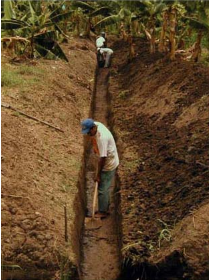
Figure 14. Beginning to clean the 50 m profile documented as Suboperation 5, looking north.
