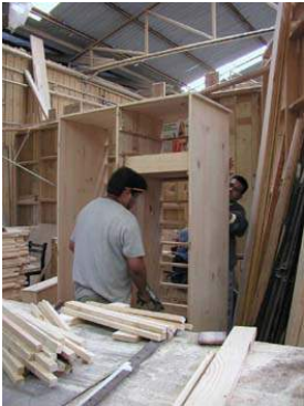
3.7 Archival Storage Construction by C.I.N.S.J.P. Photo: Gabany-Guerrero
