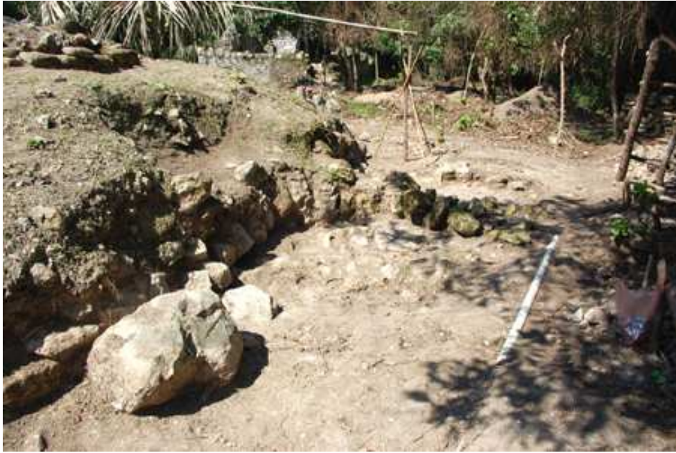
Figure 14. East end of YDL I showing a section of the shoring of slumping platform face on this side. The photo looks north.
