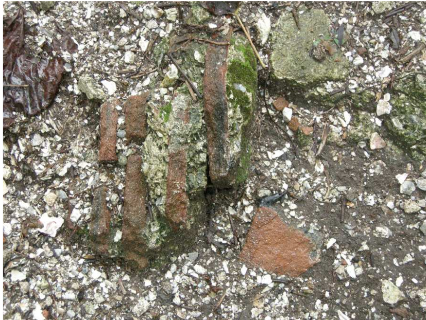
Figure 10. Brick and mortar eroding from top of Feature 196.
