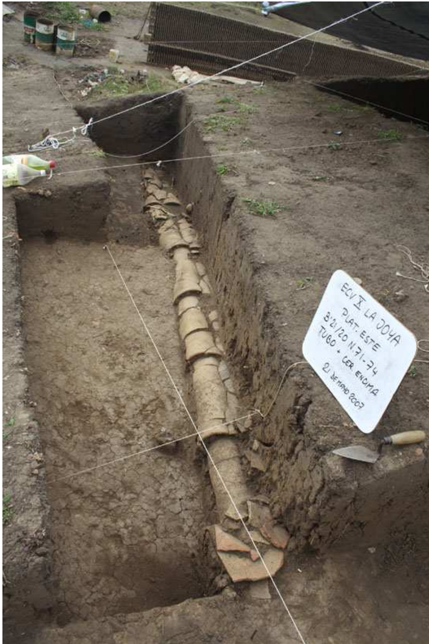
Figure 7. East Platform: drainage of ceramic tubes from the fourth building stage.
